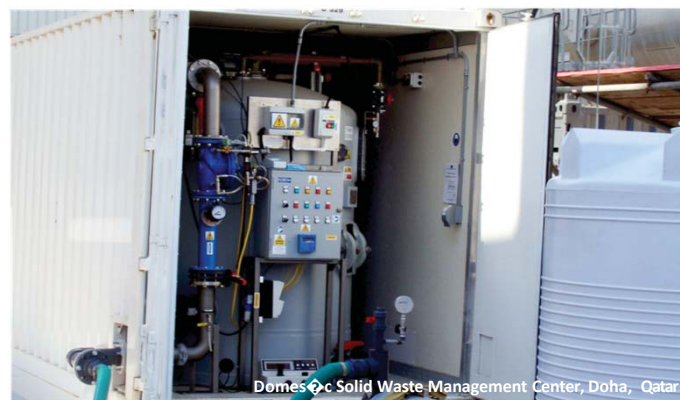
Domes Solid Waste Management Center, Doha, Qatar
